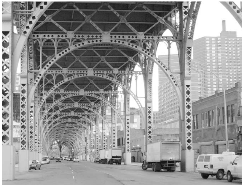
Viaduct near the historic Harlem Piers.
